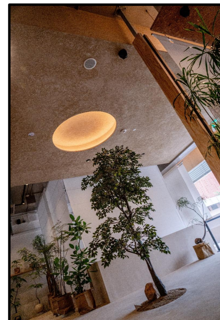
Lime Plaster on ceiling and floor
