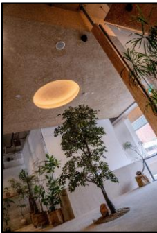
Lime Plaster on ceiling and floor
